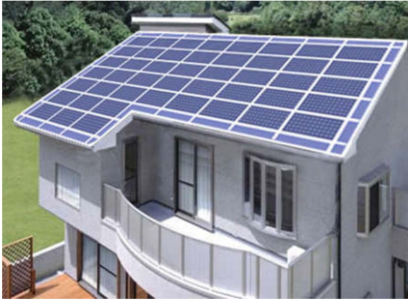
Fig. 3. Building Integrated PV system.
