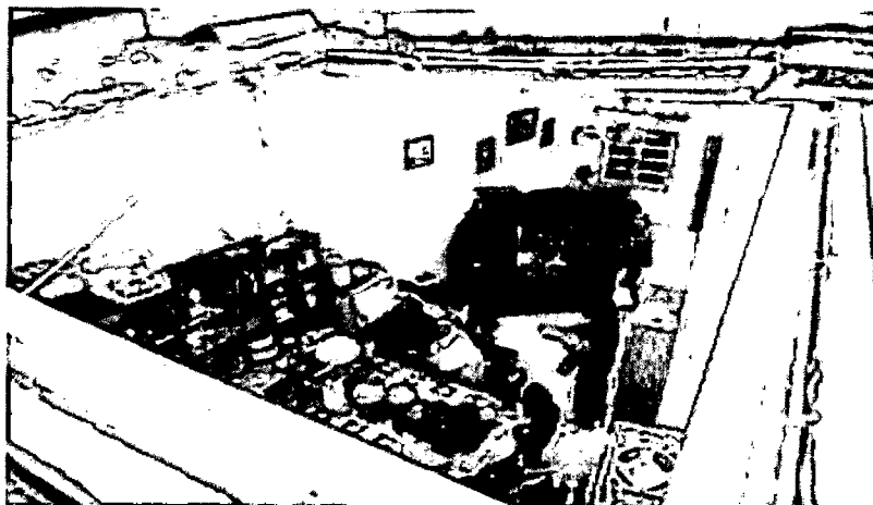
Figure 1.3 : Roof Damage (T.A. Majid et al, 2010)
