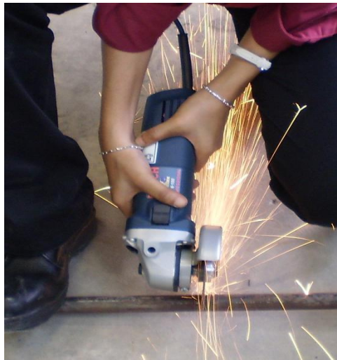
Figure 3.10: Cut material into the wanted shape
