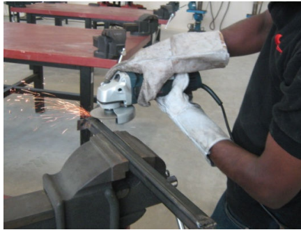
Figure 3.22: Grinding the weld parts
