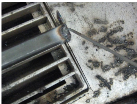
Figure 3.21: Weld the parts
