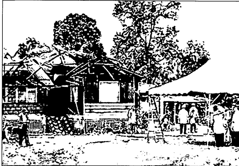
Figure 1.2: Roof Damage (2) (Utusan Malaysia, 2010)
