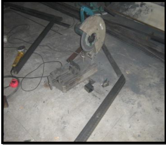
Figure 3.9: Cutting the rectangular bar with disc cutter The stainless steel bar has been cut by disc cutter to give it straight cut.
