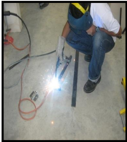
Figure 3.10: Joining the rectangular bar
