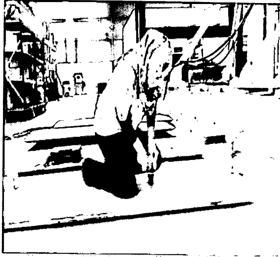
Figure 3.10: The screws tapping activity using hand-drill machine
