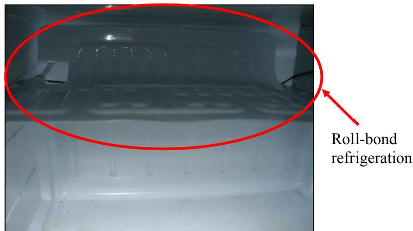
**Figure 2.6:** Roll-bond refrigeration evaporator
