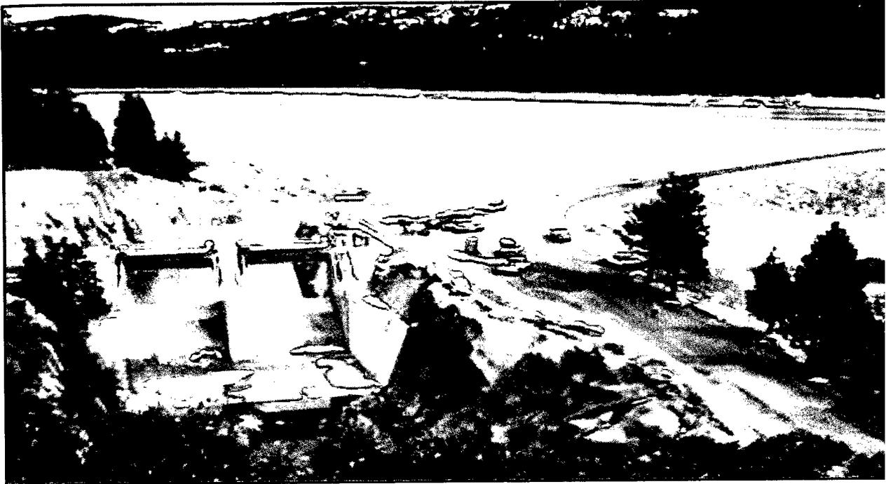
**Figure 2.3:** A spillway bucket of Anderson Dam, California (terramaterang.com,2007)
