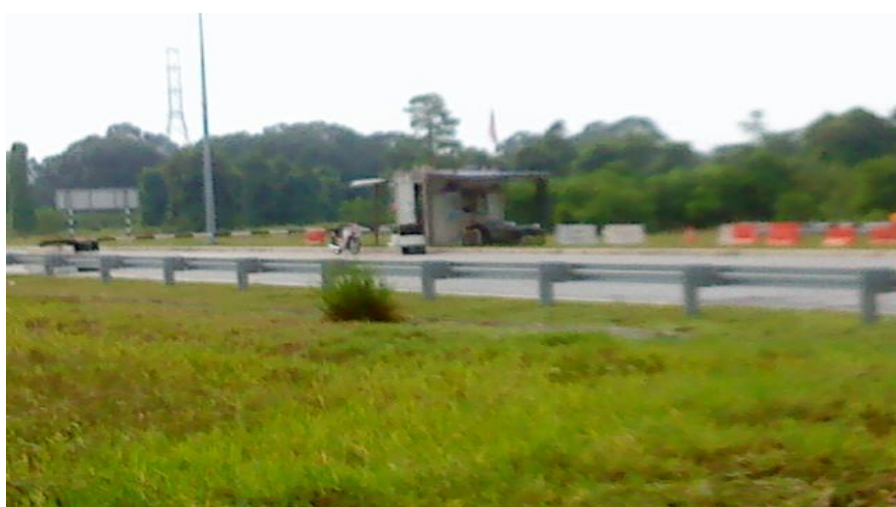
Figure 5.4: Main entrance of Tanjong Agas oil and gas complex
