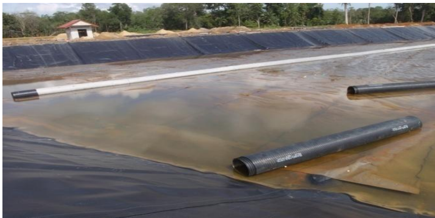
Figure 3.3: Sanitary landfill under construction
