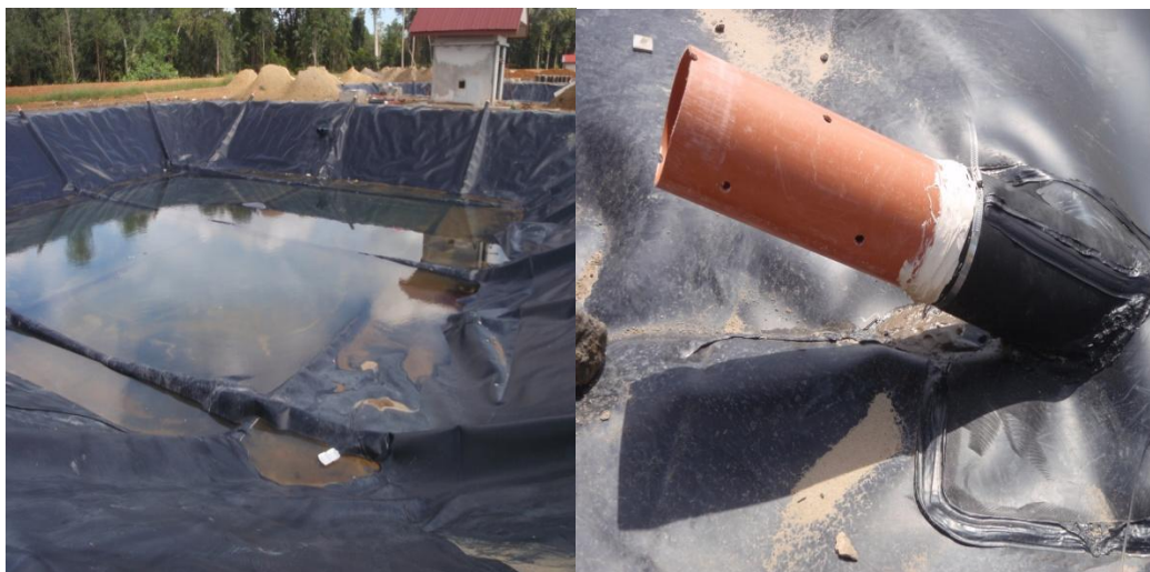
Figure 3.4: Leachate treatment ponds
