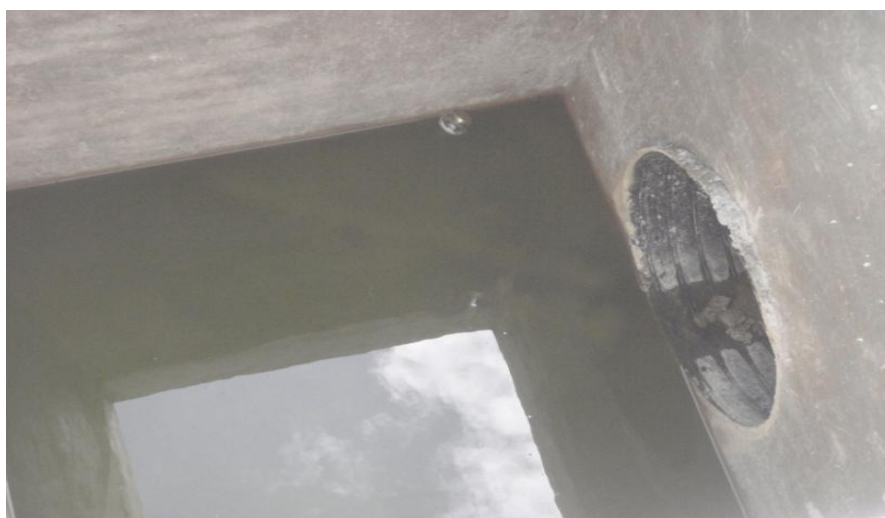
Figure 3.7: Leachate duct and pre-container
