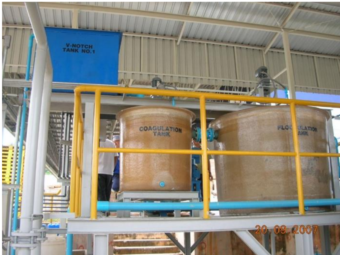
Figure 2.7: Coagulation and Flocculation Tank (Dynamic-des.com, 2014)
