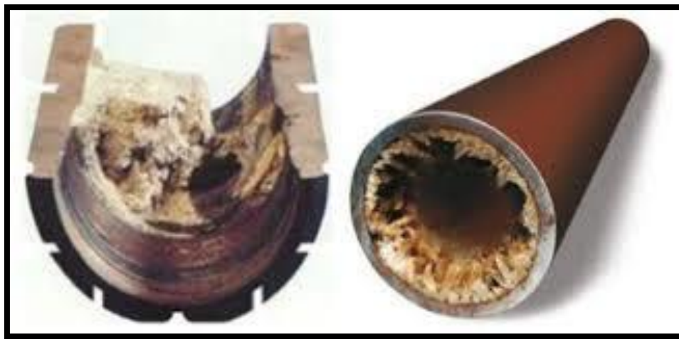
Figure 2-1: Picture of sulphate scales formed in a pipeline.
