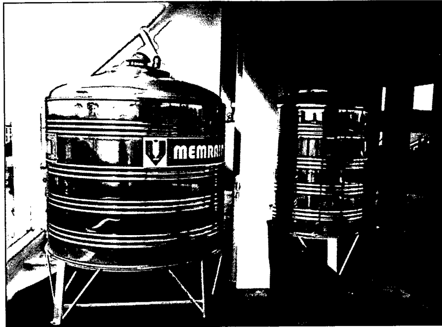
Figure 2.1: Collected rainwater tank and treated water tank
