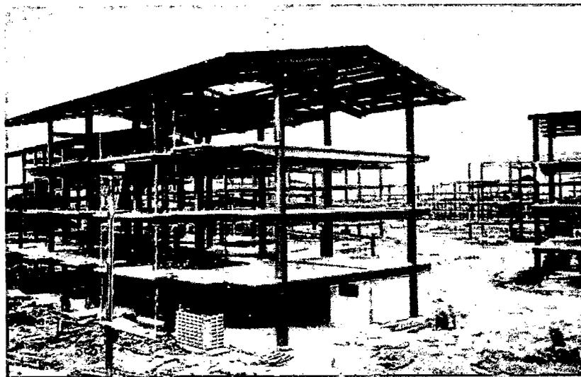
**Figure 2.4: Steel frame system**
