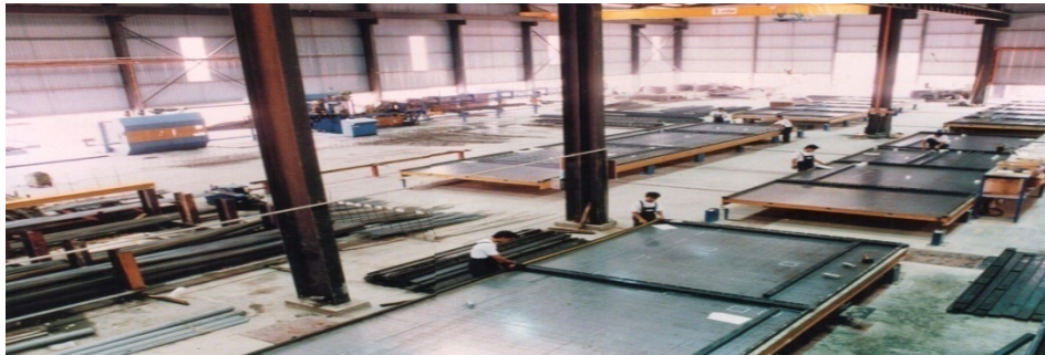
Figure 2.8: Do the formwork for pre-cast component
