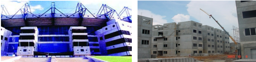
Figure 2.1: Pre-cast concrete framing system
