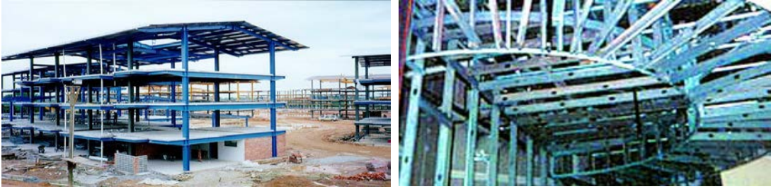
Figure 2.3: Steel framing system
