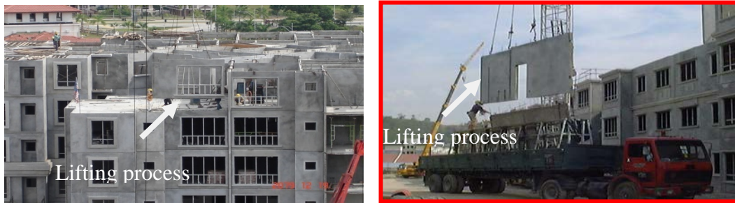
Figure 2.15: Example of lifting process
