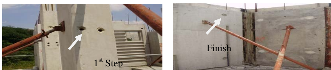
Figure 2.19: Step of grouting process used pumped method
