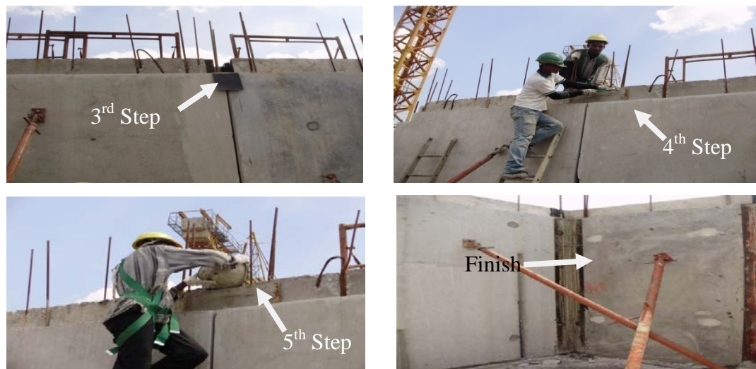
Figure 2.18: Step of grouting process used placement method
