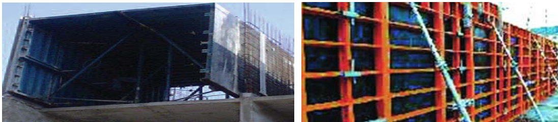
Figure 2.2: Steel Formwork Systems
