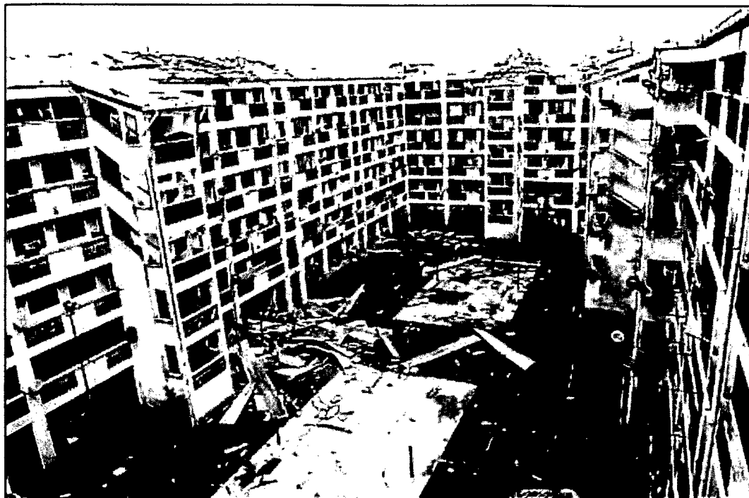
Figure 2.2: Apartment Roof Damaged Cause by Thunderstorm, (Nadirah, 2012).
