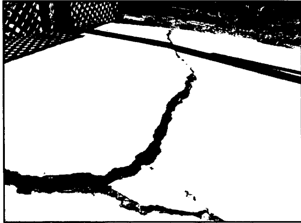
Figure 2.2 : Cracking of the floor because the low quality of material
