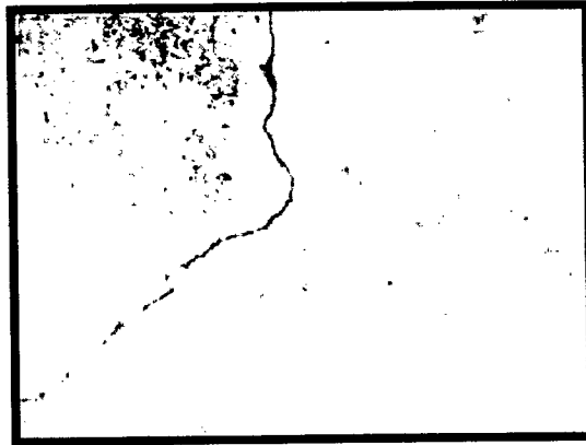
Figure 2.2: Hairline cracking
