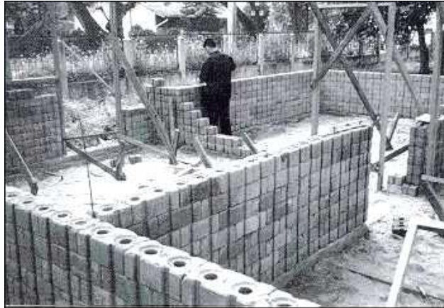
Figure 2.1 : The Thai interlocking block (Kintingu , 2009 )
