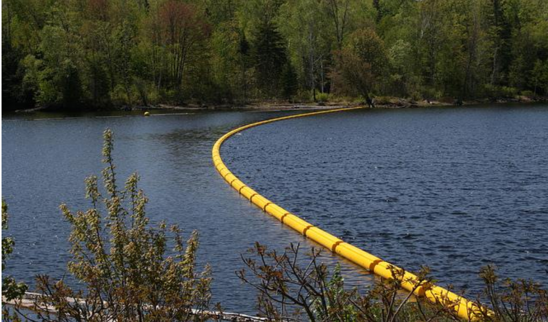
Figure 1.3: Floating boom was placed in the middle of the river or lake to block and capture the debris or trash.
