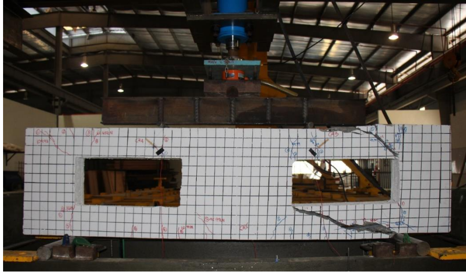
Figure 4.9: Crack pattern after failure for beam US-BRO
