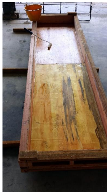
Figure 3.2: Formwork of beam specimen
