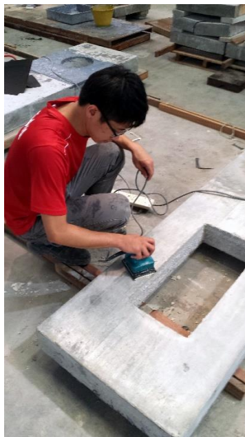
Figure 3.11: Polishing concrete surfaces using polish machine
