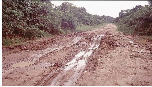
Figure 2.1 Rutting of pavement
