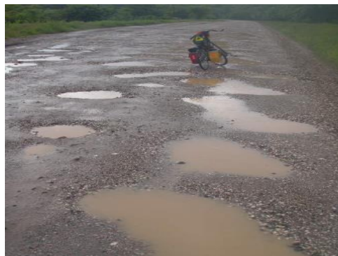
Figure 2.2 Potholes on road pavement.
