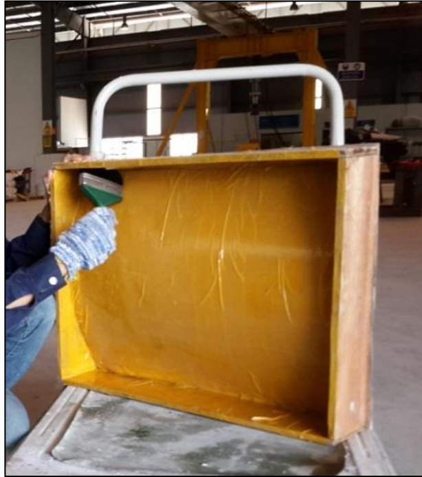
Figure 3.7 : Oiling works on formwork.
