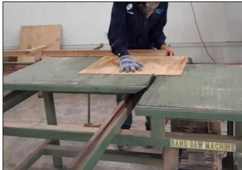
Figure 3.4 : Plywood cutting for arch slab formwork.
