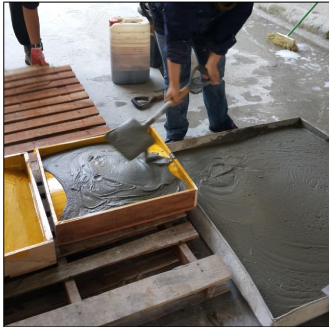
Figure 3.11 : Pouring stage of arch slab
