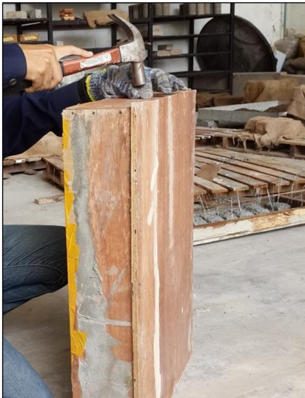
Figure 3.5 : Formwork preparation for arch slab.
