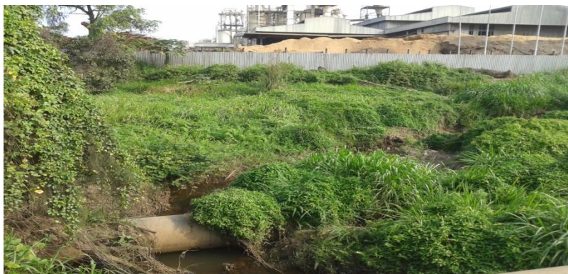
Figure 4.15: Wooden Industry near to station 1
