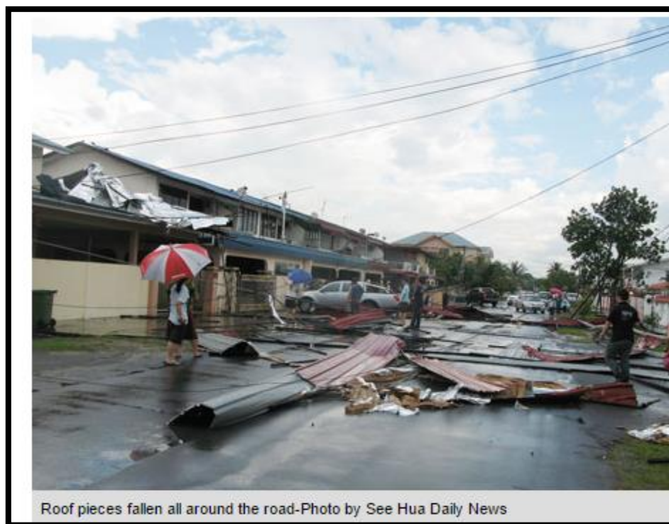
Figure 1.2 Damaged in Sibuan
