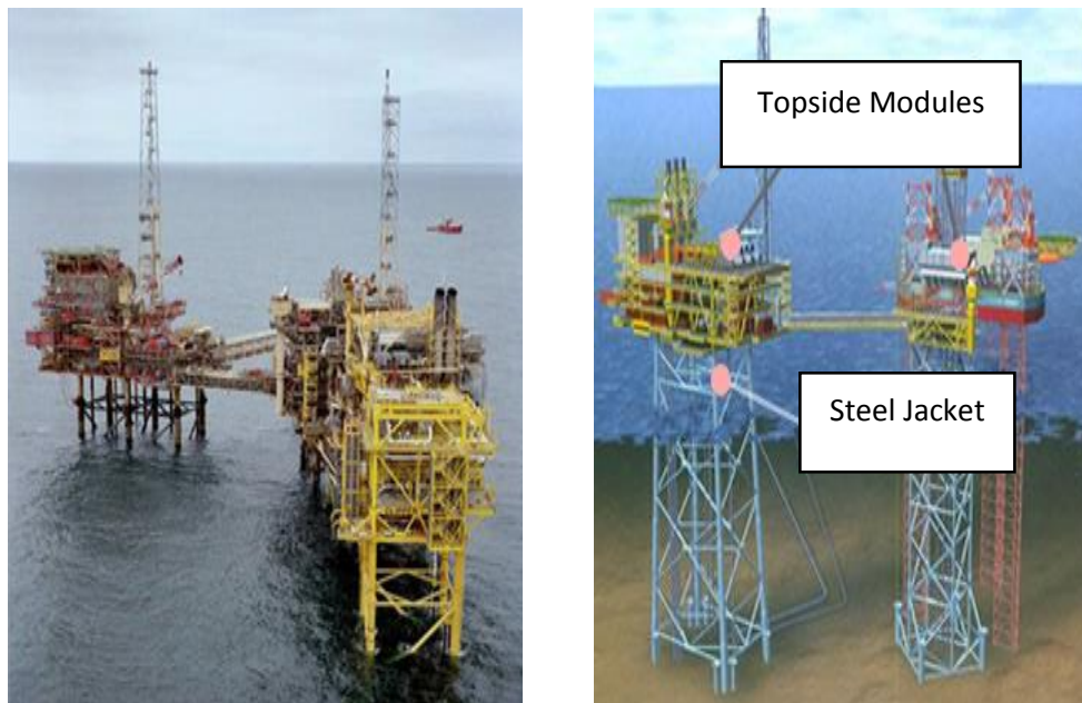
Figure 2.1: Real model on offshore jacket platform
