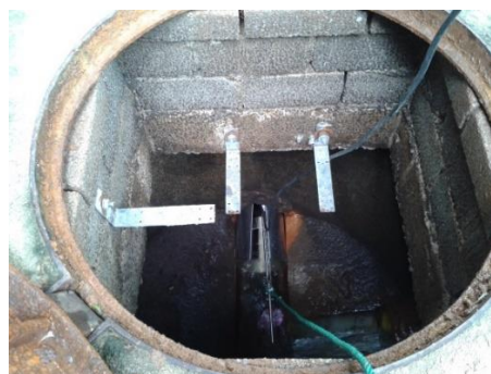
Figure 3.13: Mounting ring that fixed the sensor
