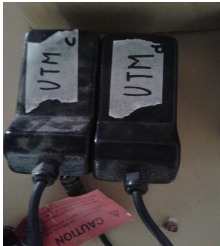
Figure 3.10: Lead Acid Battery from UTM
