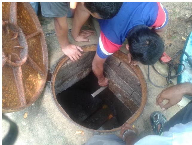
Installation of hanger steel plate in manhole by contractor
