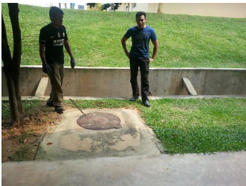
Figure3.4: Manhole 6 Site Visit
