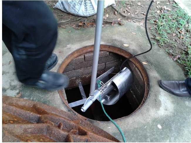
Install the sensor into manhole by using mounting ring
