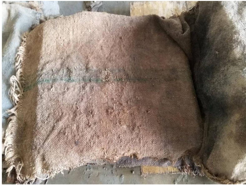
Figure 3.10: Curing with wet sack
