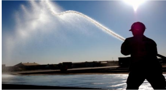
Figure 2.6: Sprinkling water method of curing
