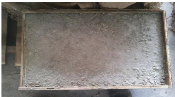
Figure 3.18: Hardened slab before dismantling from formwork
