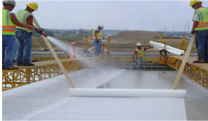
Figure 2.3: The curing of concrete by membrane curing method
