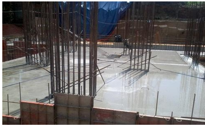
Figure 2.4: The curing of concrete by ponding method
