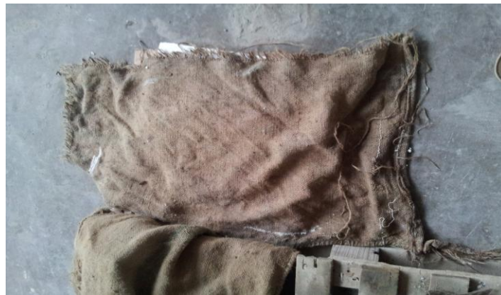
Figure 2.7: Wet covering is overlapped onto the concrete surface for curing
