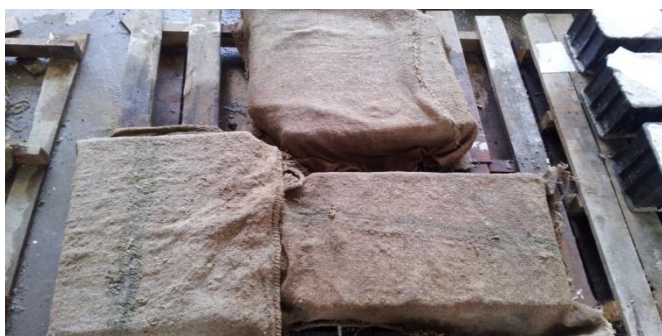
Figure 3.19: Curing of concrete using wet gunny sack
