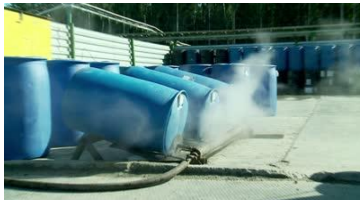
Figure 2.5: The steam curing method applied the heat to the concrete
