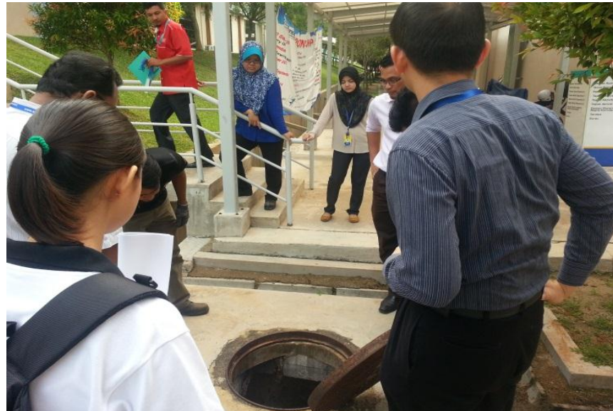
Figure 3.10: Selected manhole (MH 07)
