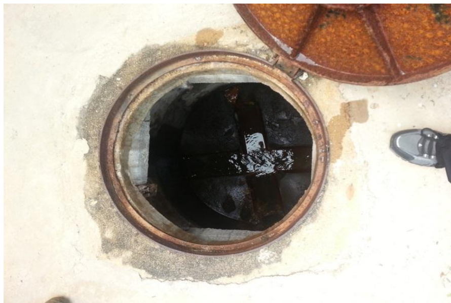
Figure 3.11: Sewer pipeline located under the manhole
