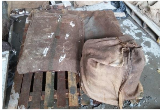
Figure 3.8: Curing process using wet gunny bags
