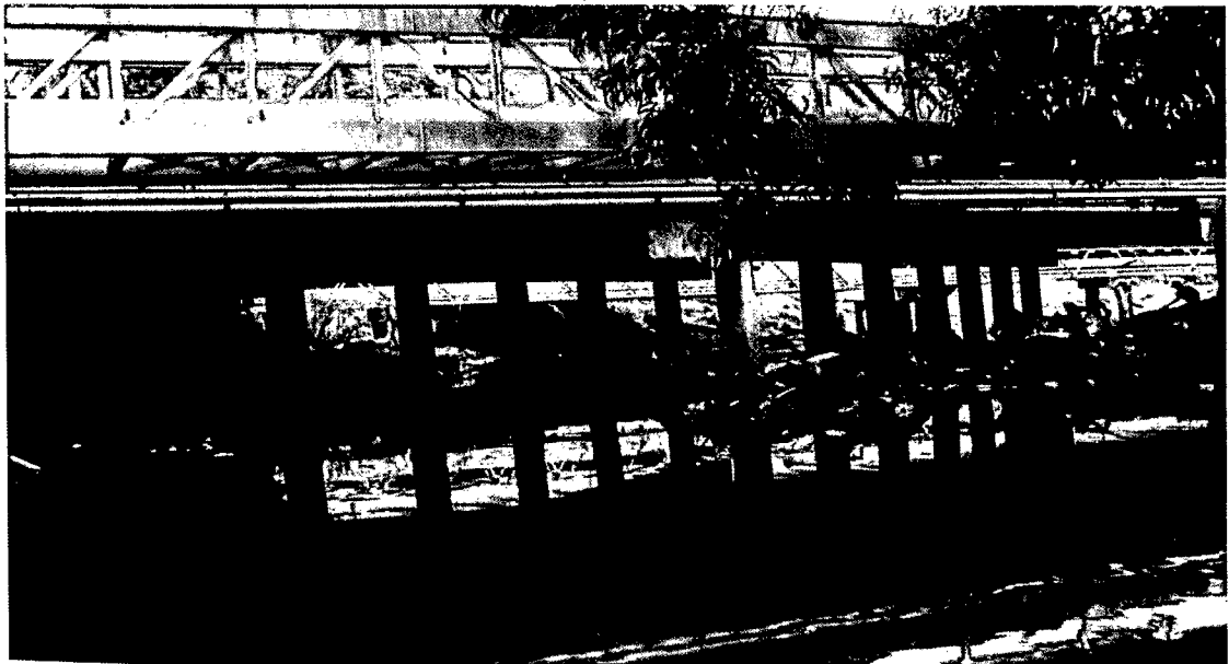
Figure 1.1: Bridge of Galing River, Kuantan
