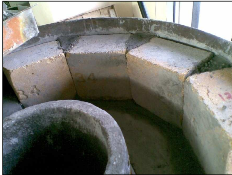
Figure 3.17: Arrangement of firebrick before finishing
