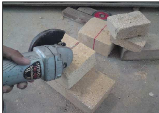
Figure 3.16: Cutting the firebricks
