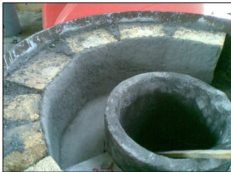
Figure 3.18: Finishing on the surface of wall
