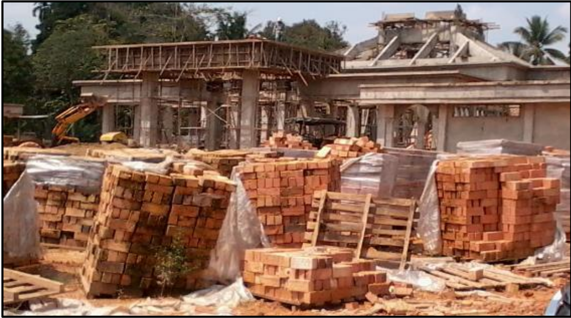
Figure 1.2: Masonry units used in construction site
