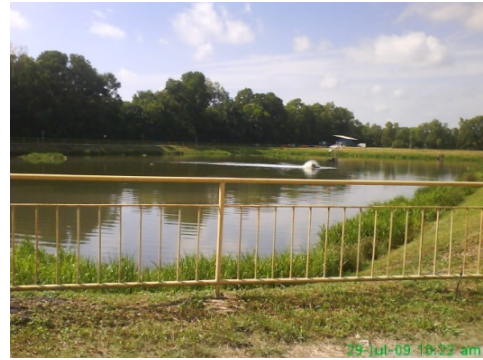
Figure A-10 : Sewage treatment plant
