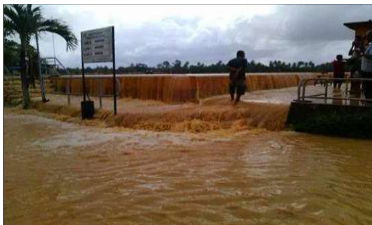
Figure 2.7 The water overflows the riverbank at Dataran Air Muleh, Pasir Mas
