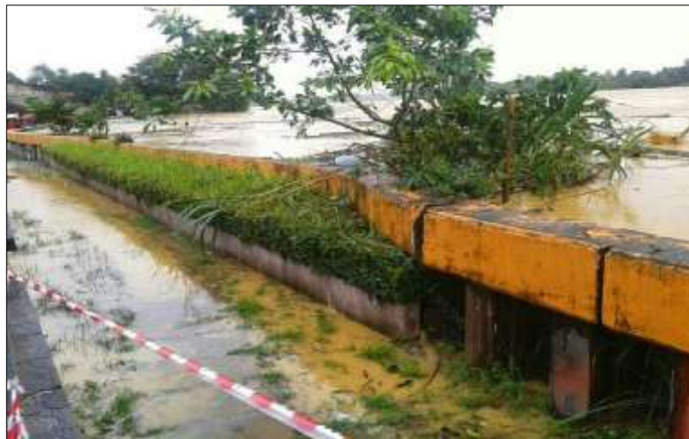
Figure 2.6 The riverbank area at Dataran Air Muleh, Pasir Mas
