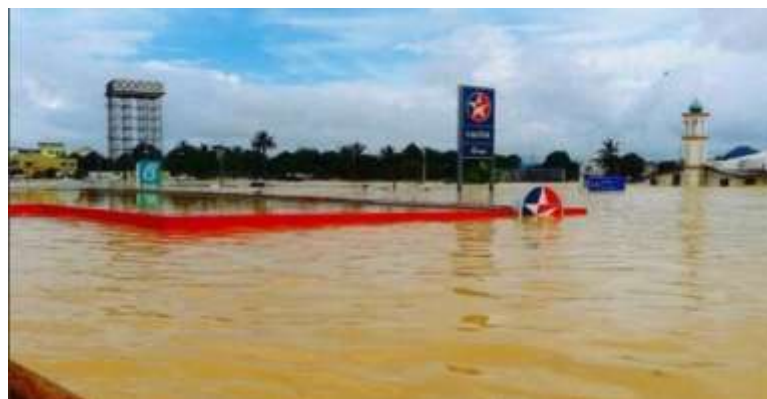
Figure 2.1 Pam station at Kuala Krai under water during flood
