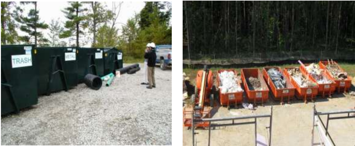
Figure 2.2: (a) and (b): Example of Construction solid waste separate at the construction site
