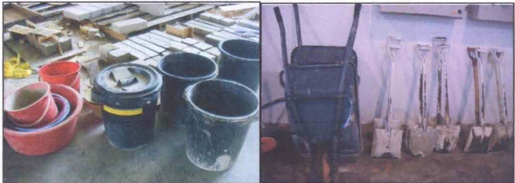
Figure 3.10 : Tools and equipment used during concrete batching
