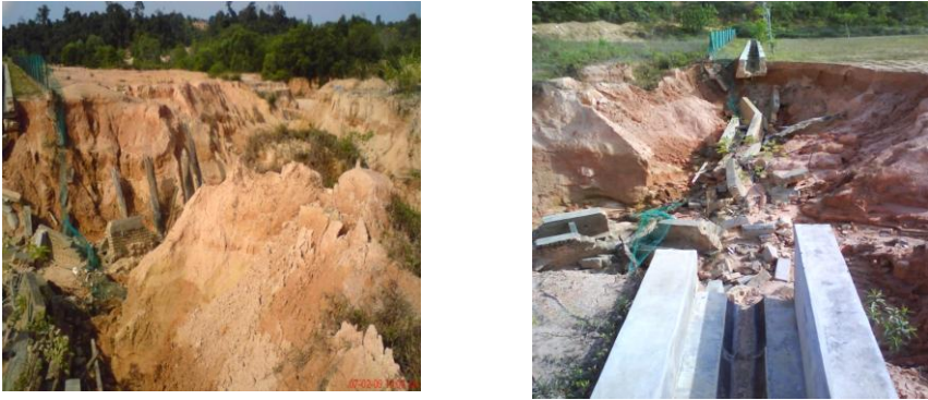
Figure 1.1: The property damage because of the soil collapse
