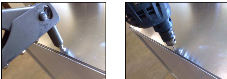
Figure 3.9.1(d): Drilling and Riveting Process
