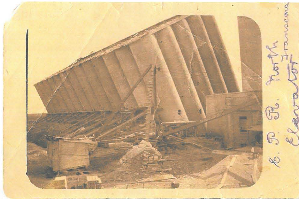
Figure 1.4: Failure at Transcona Grain Elevator
