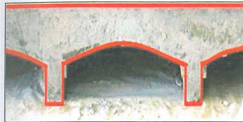
Figure 2.10: Arch concrete slab system model
