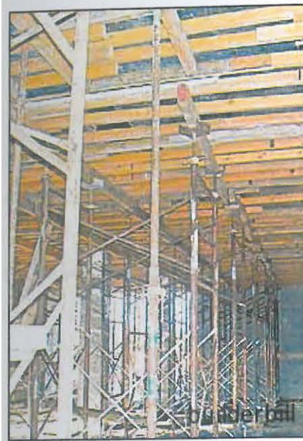
Figure 2.6: Traditional slab formwork
