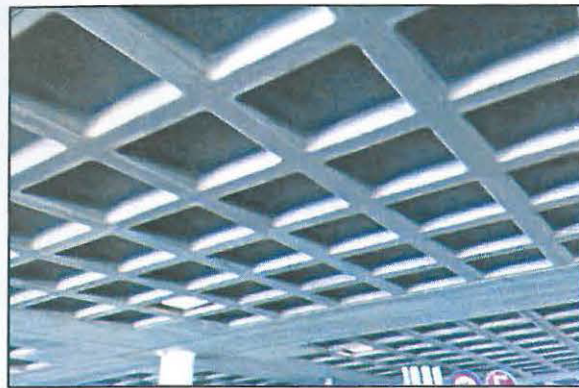
Figure 2.3: Waffle slab
