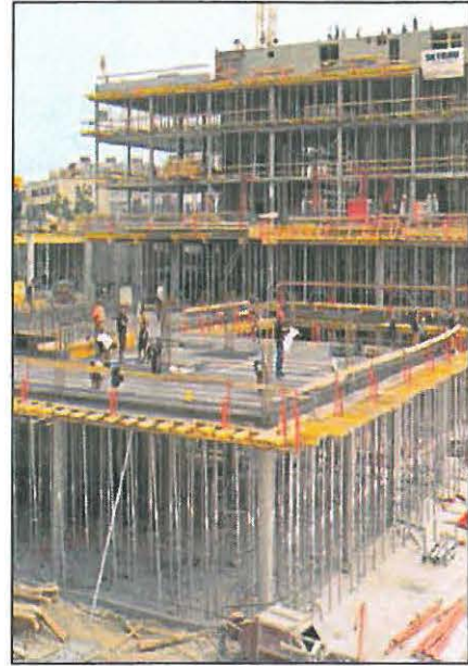
Figure 2.7: Metal beam slab formwork
