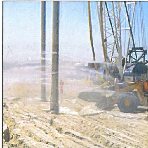
Figure 2.2 Vibro-compaction
