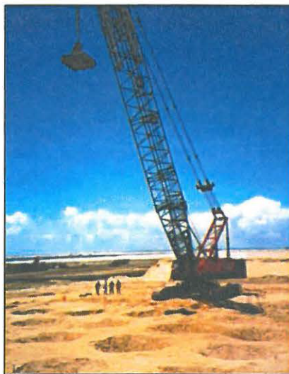
Figure 2.1: Crawlers Dynamic Compaction Machine
