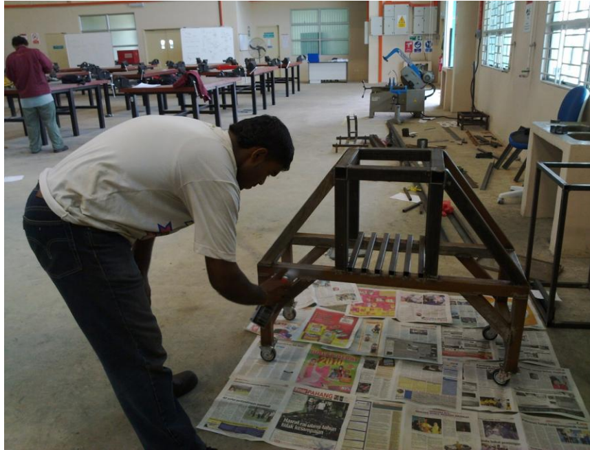
Figure 3.29: The finished test rig is being sprayed to ensure it does not rust.
