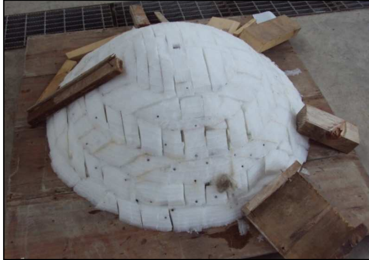
Figure 3.13: Mould after adding the polystyrene
