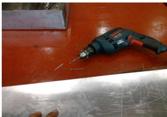
Figure 3.15: Using hand drill to drill holes for rivet
