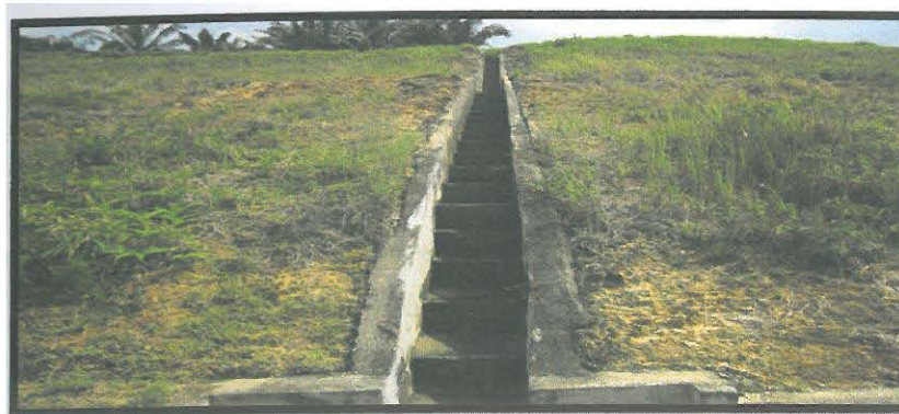
Figure 2.1: Stepped channel that usually seen in hill area.
