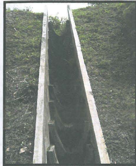
Figure 2.7: Parabolic stepped channel
