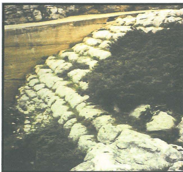
Figure 2.2: Old stepped weir (dam) in Akarnania, Greece B.C. 1300
