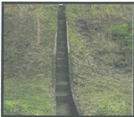
Figure 2.6: Rectangular stepped channel
