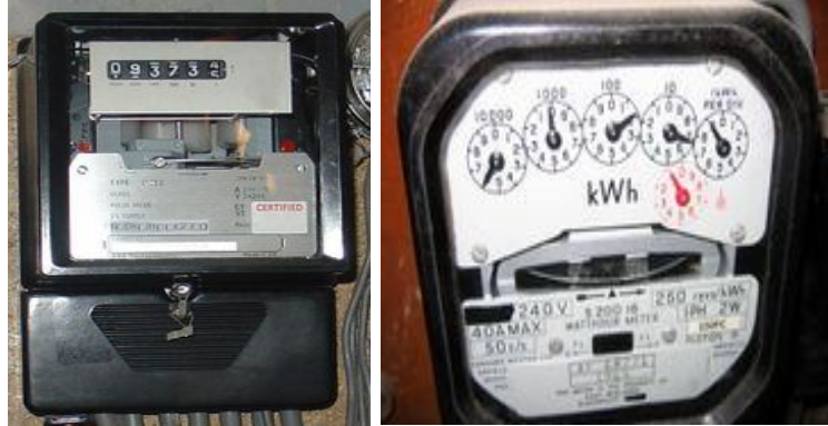
Figure 1.2: Electromechanical Induction Meter
