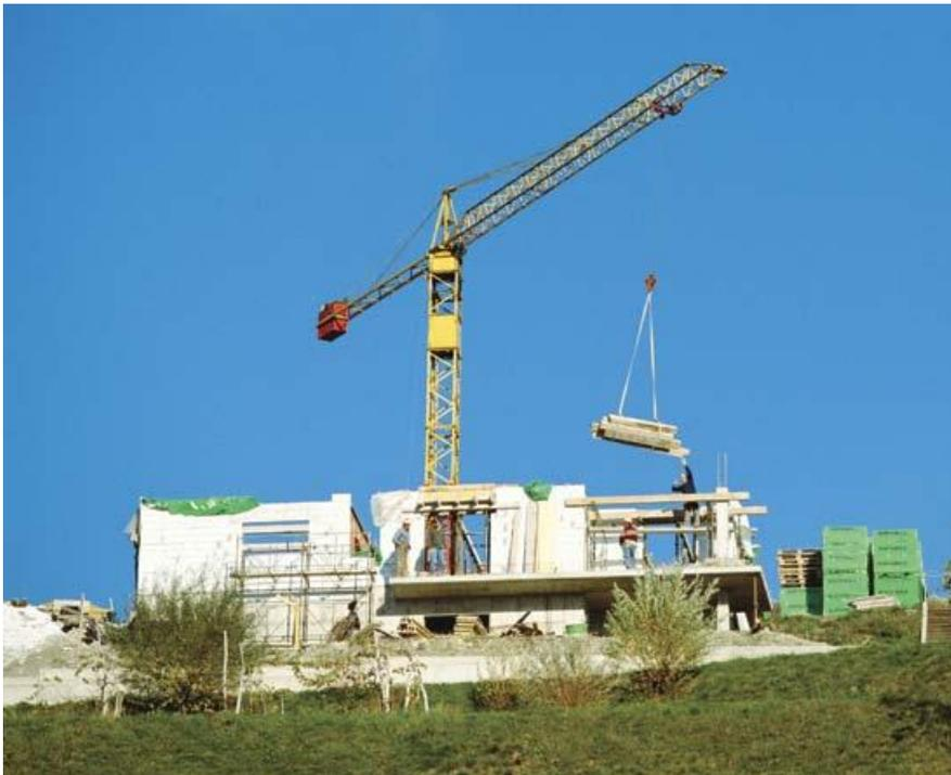
**Figure 1.1:** Rotary Crane
