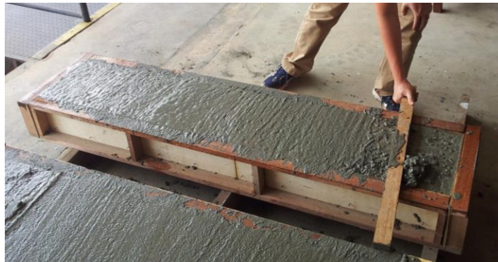
Figure 3.24: Surfacing the beam
