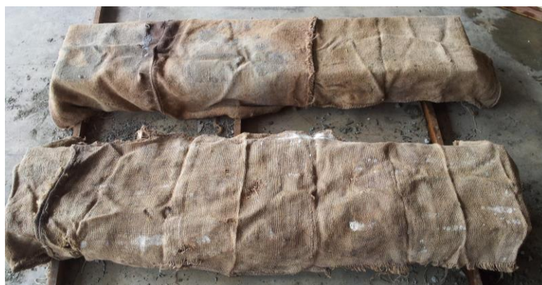
Figure 3.29: Gunny bags were used to cover beams for curing
