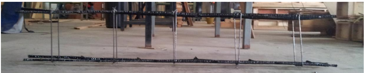
Figure 3.11: Bamboo used as main reinforcement
