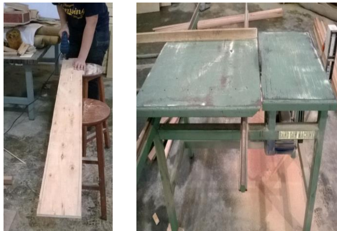
Figure 3.17: Machineries used to cut plywood and wooden planks
