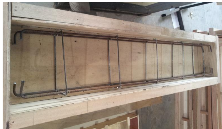
Figure 3.14: Steel reinforcement was placed in formwork
