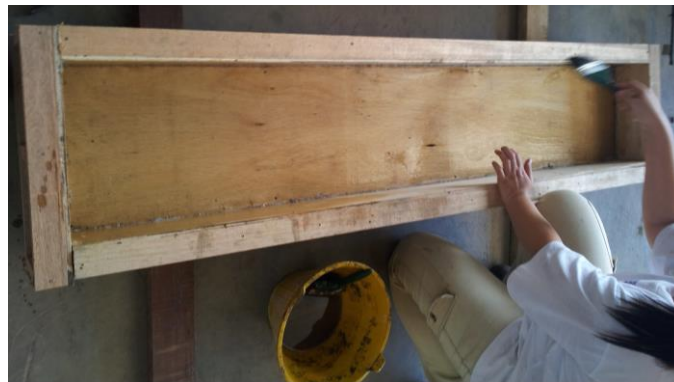
Figure 3.21: Formwork must be applied with grease before pouring concrete
