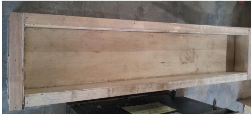
Figure 3.20: Formwork must be free from impurities
