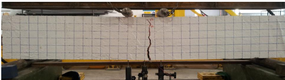
Figure 4.35: Crack pattern for bamboo reinforcement (BR)
