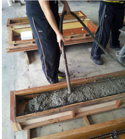
Figure 3.23: Vibrating concrete using hand-held vibrator
