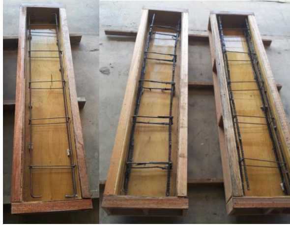
Figure 3.22: Reinforcements were placed in formworks
