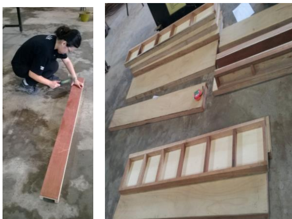
Figure 3.18: Formwork fabrication works in progress
