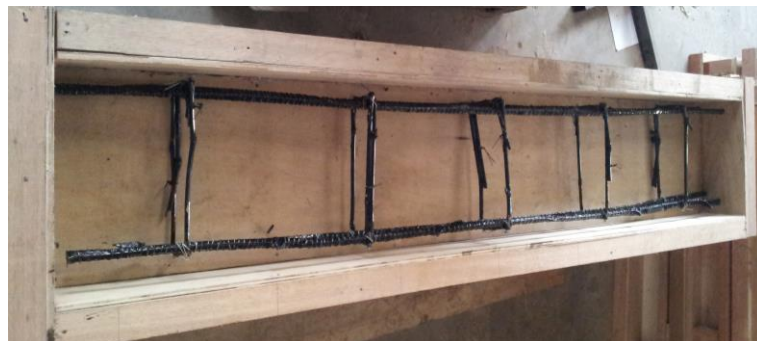
Figure 3.12: Bamboo reinforcement were placed in formwork
