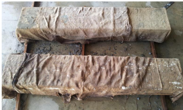
Figure 3.30: Wetted gunny bags for concrete curing
